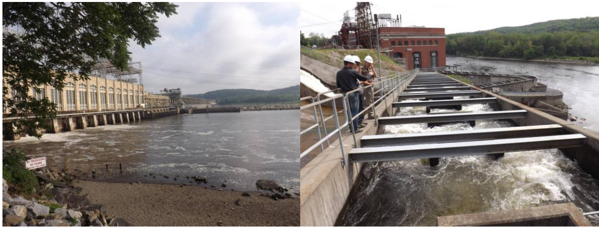
Figure 3: View of Conowingo powerplant and the fish lift on the Susquehanna river (left) and the fish pass of Cabot Station on the Connecticut river (right)
