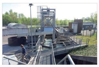
Fishway with monitoring station at the Gambsheim dam, the second obstacle for migrating fish in the Rhine
