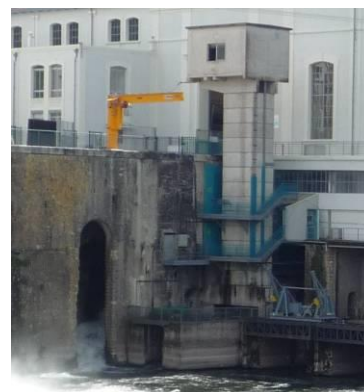
Pic. 28 : The fish lift at Tuilières
